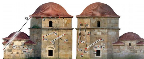
Figure 3: The pairs of defined feature points used for data accuracy verification [16].
